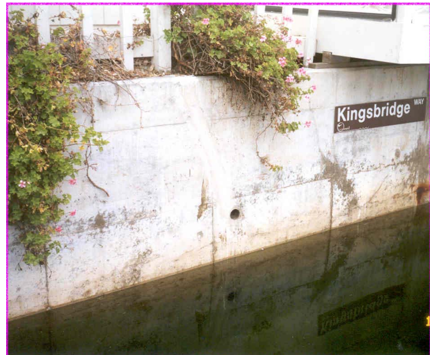
After repair with urethane grout
