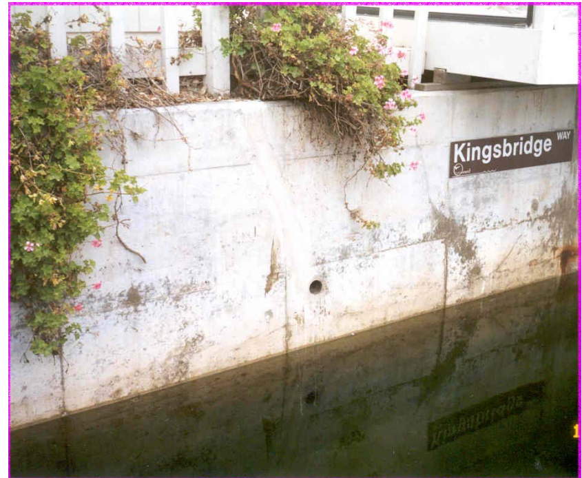
After repair with urethane grout
