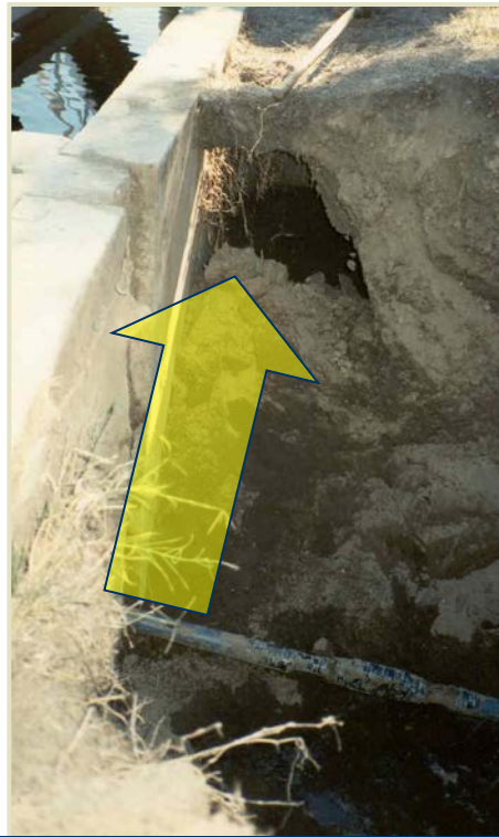
Excavate to uncover extent
