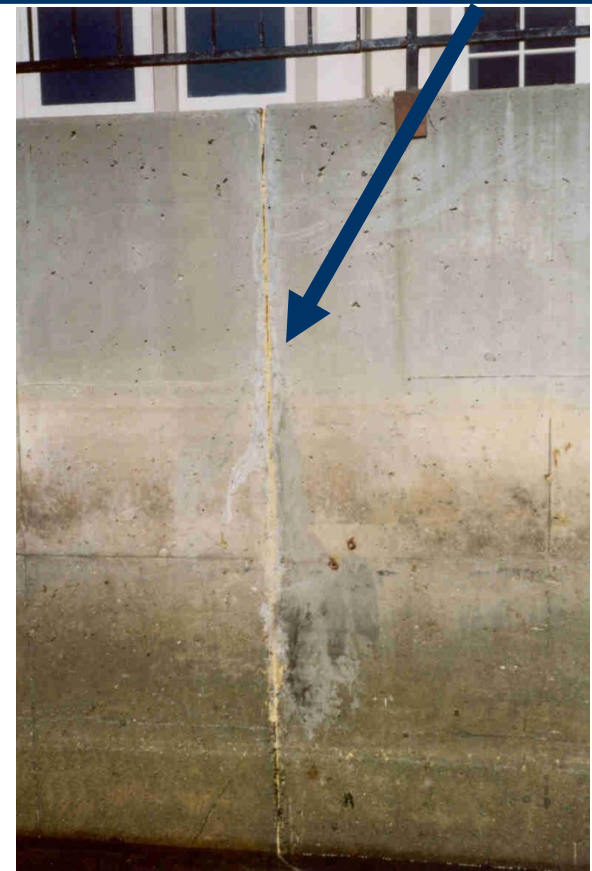
Zurn Wall joint repaired and sealed with urethane grout
