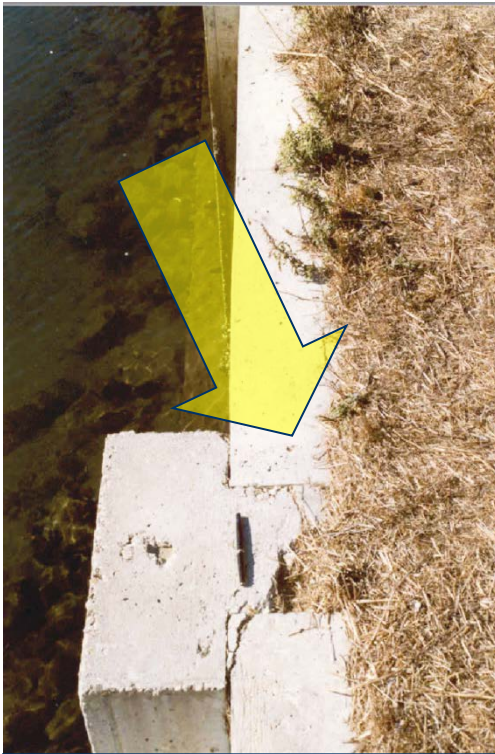
Small indication at surface
